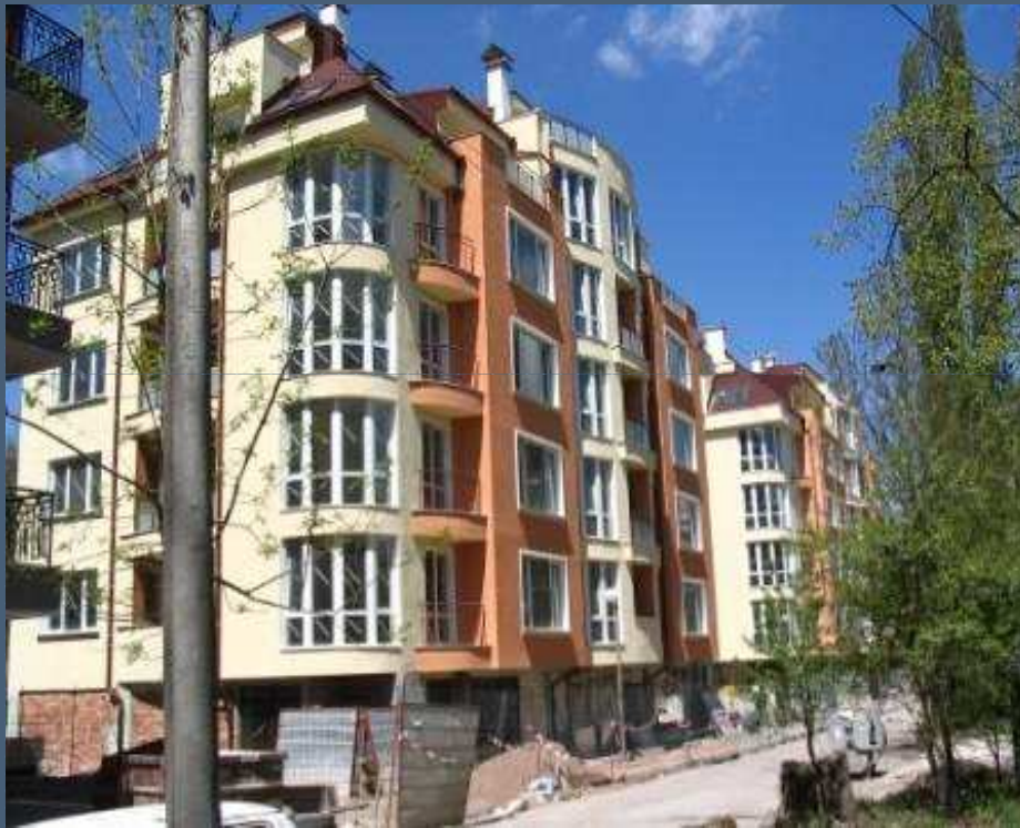
Building "A" (24.10m/11.50m)
